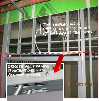
Typically, the drawings and/or specifications show just a bottom track for the door header...generally, this is **NOT** enough based on the capacity of the bottom track.
